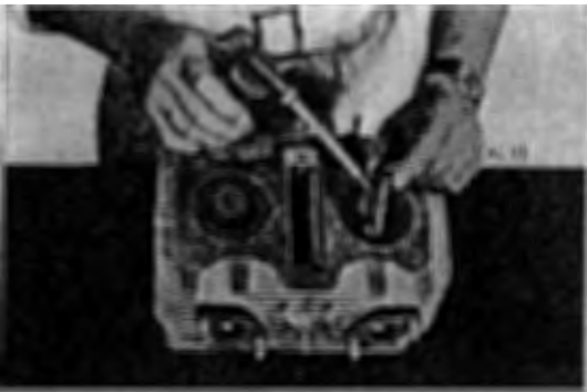
Fig. 3.35 Oiling the valve stem
