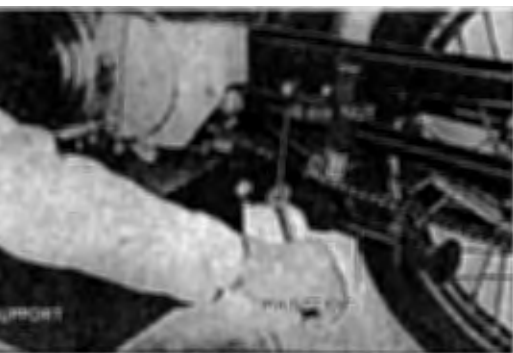
Fig. 4.47 Removing stand
